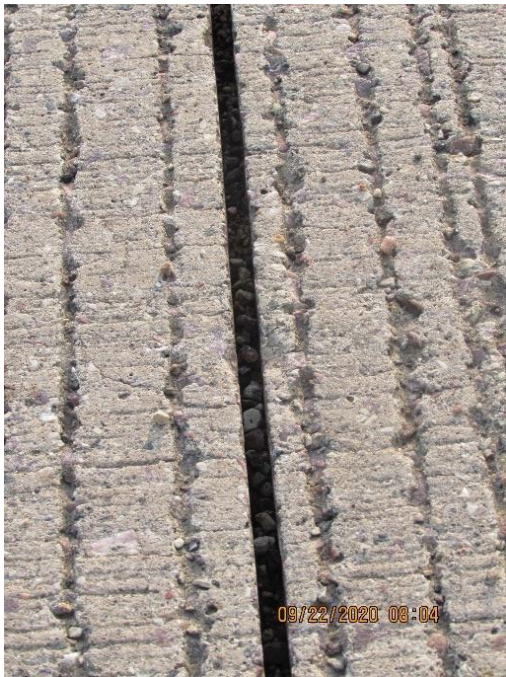
Figure 21. Another source of incompressibles showing small aggregate popped out from concrete surface and transverse tines (site # 4).
