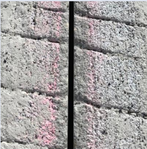
Figure 4 Photo of Media Blasted Joint
