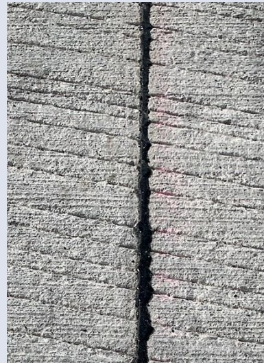
Figure 5 Properly Filled Narrow Joint
