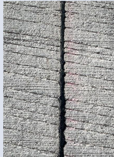
Figure 5 Properly Filled Narrow Joint
