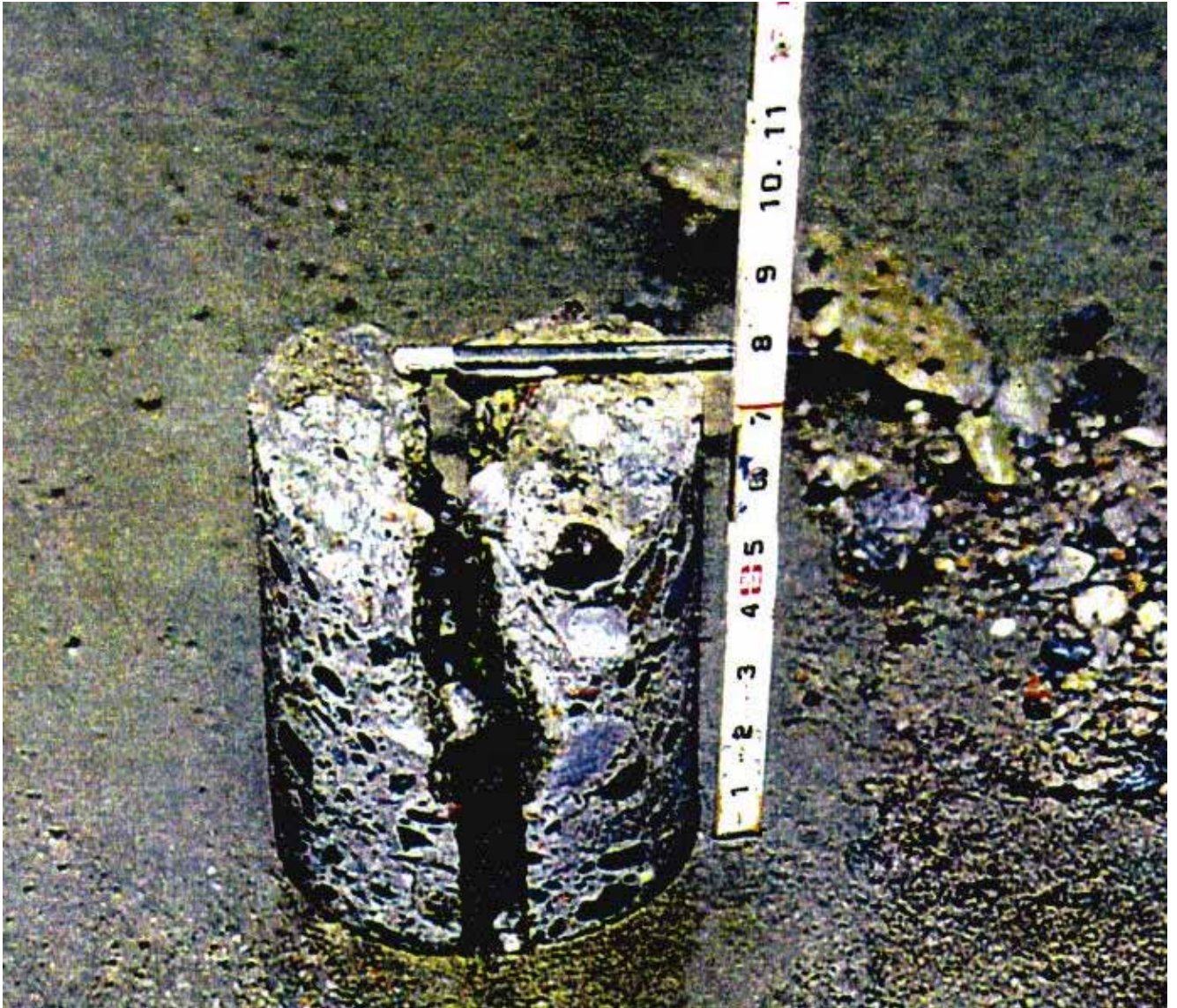
Print 5. Core of original sealed joint at 21 years of age -- 24 meter joint spacing. Considerable distress. (Core is top side down)
