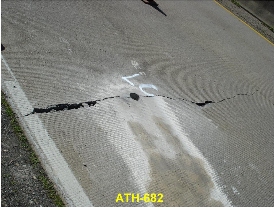
Figure 9. The coring site along a mid-slab crack on PCC pavement on State Route 682 in Athens County, Ohio. Photograph taken in 2009.
