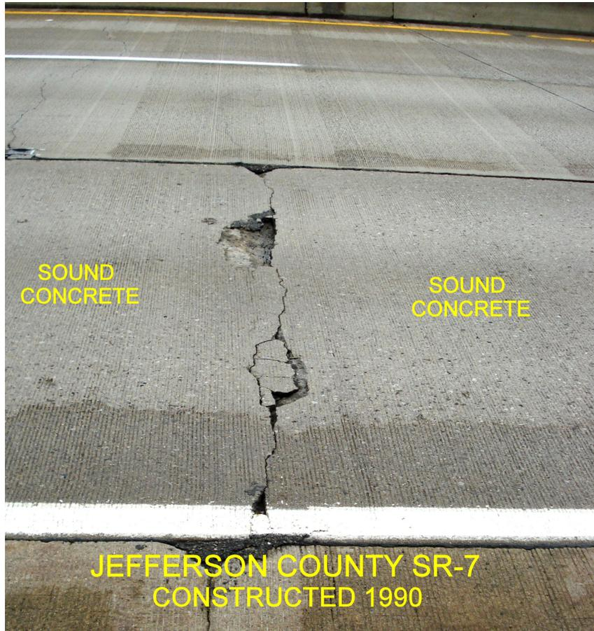
Figure 11. A mid-slab crack on the Jefferson County, Ohio State Route 7 pavement showing Type 3 cracking and spalling distress (Photographed in 2009).
