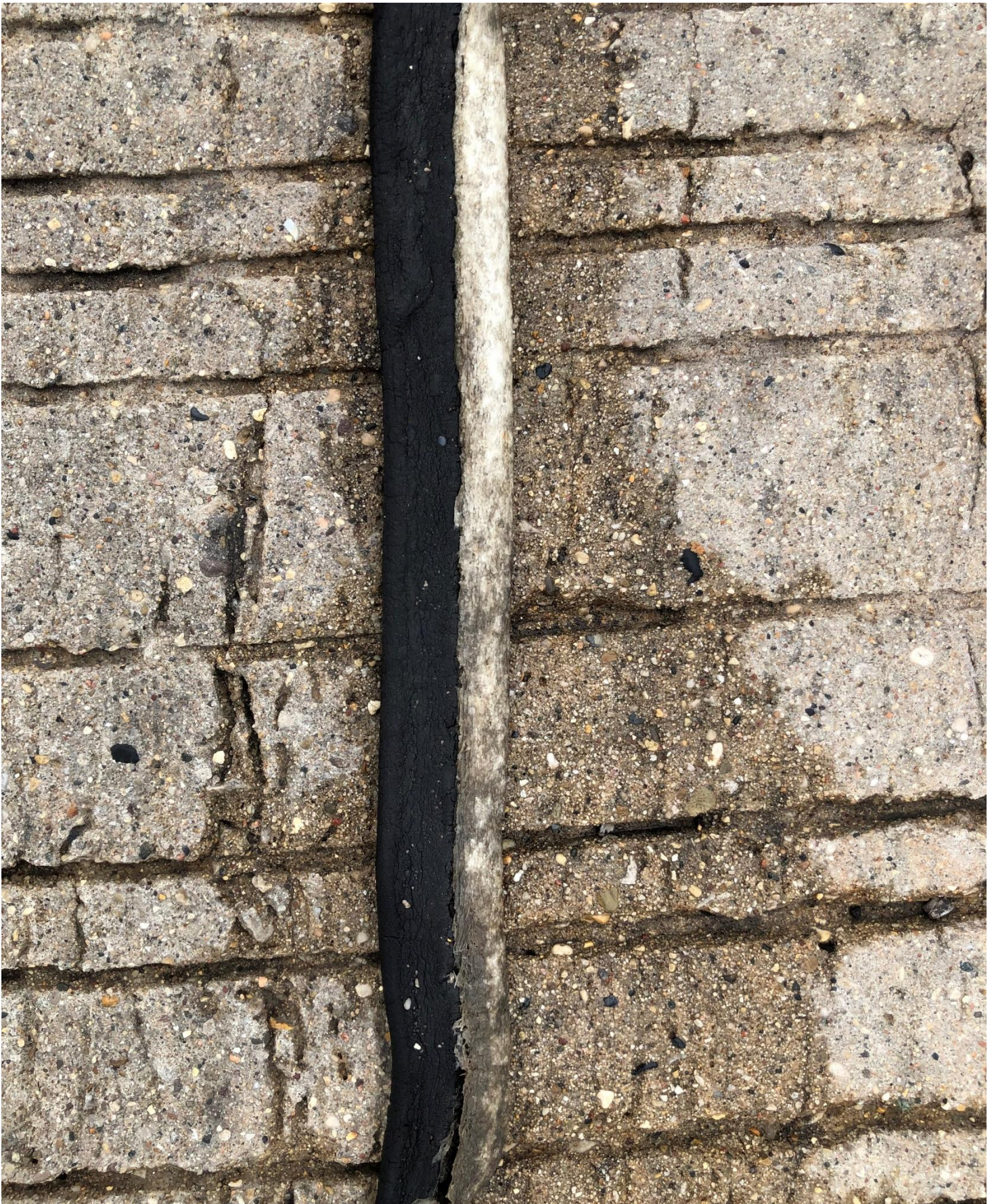
Figure 1-2 Backer Rod Floating Out from Bottom
