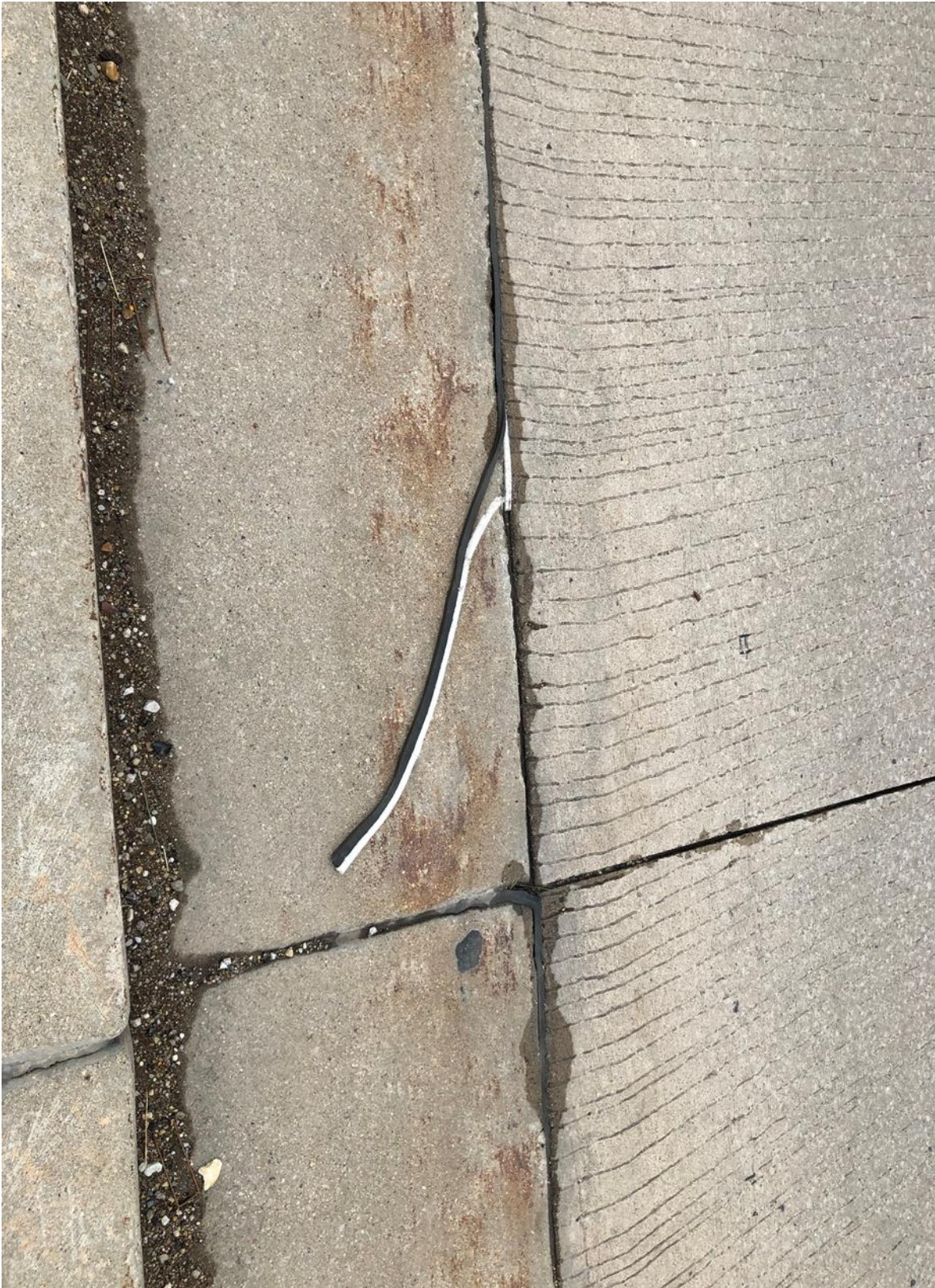
Figure 1-5 Note That Backer Rod Continues to Bonds to the Sealant
