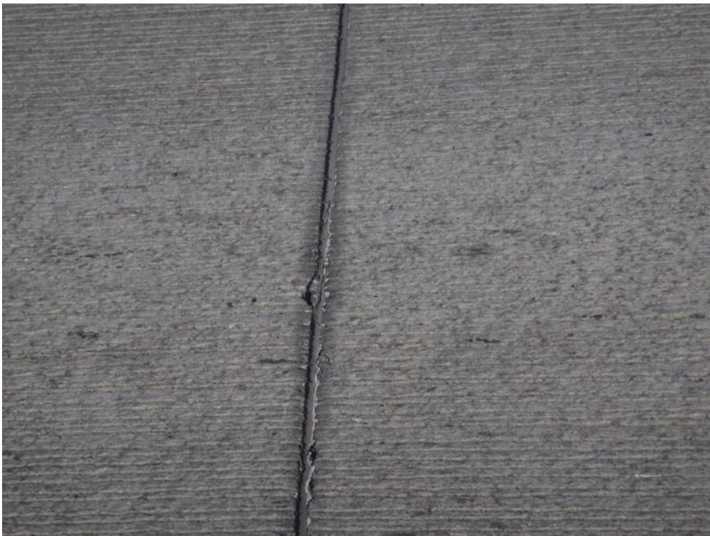
Figure 13 Silicone Sealant Wear from Tires on Old Sealant
