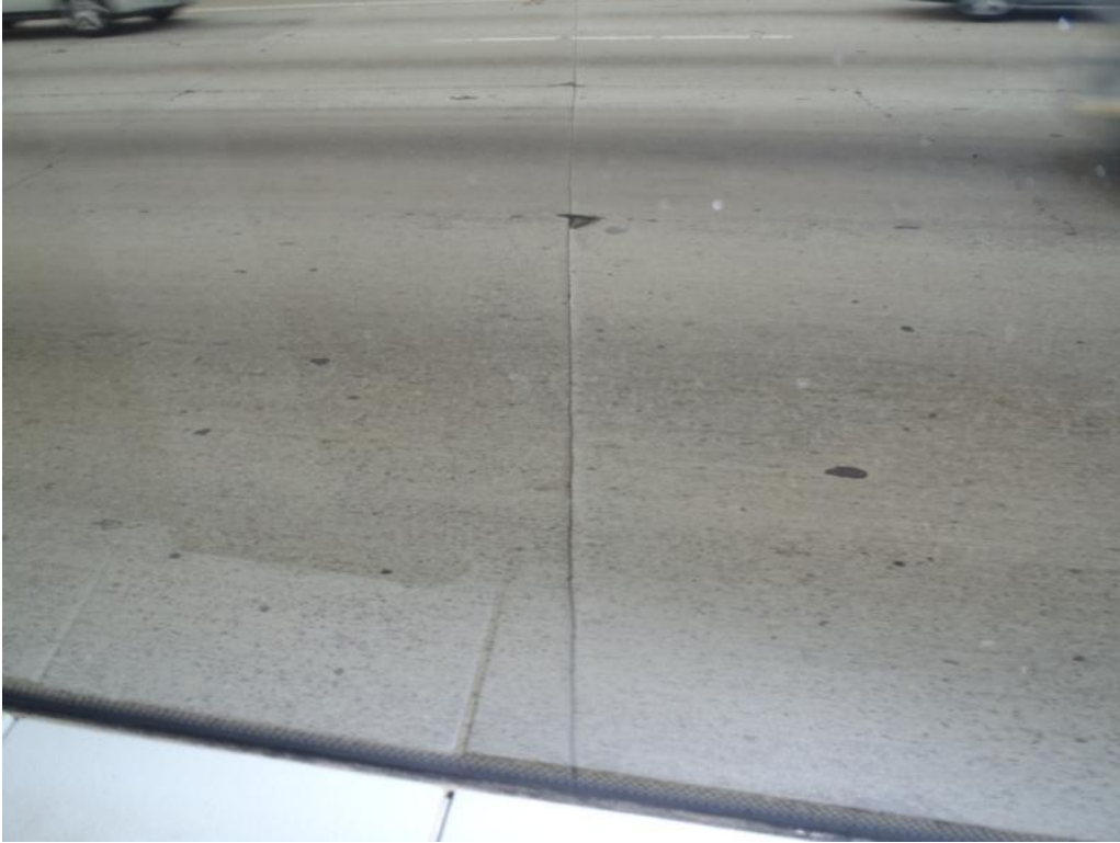
Figure 20 Tape Insert Joint
