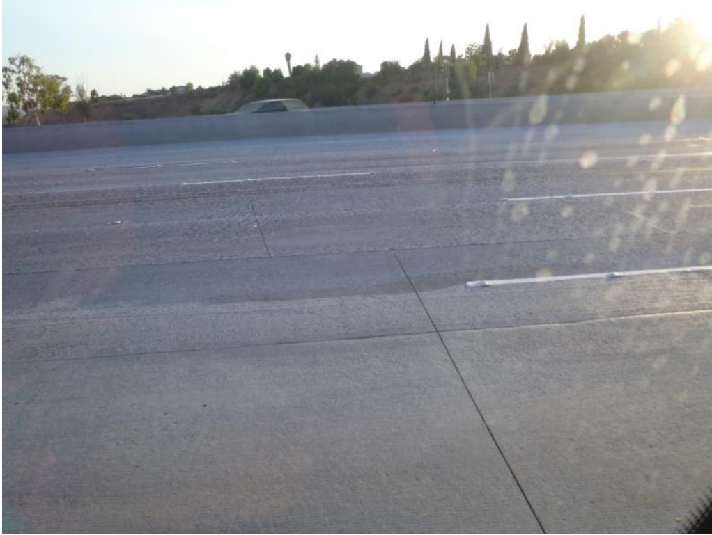
Figure 18 Misaligned Joints
