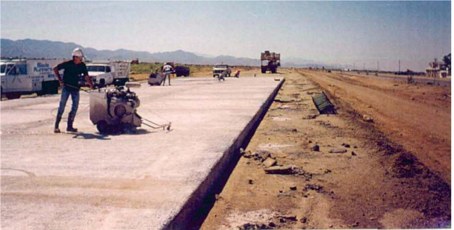
Figure 3-5 Sawing Transverse Joints
