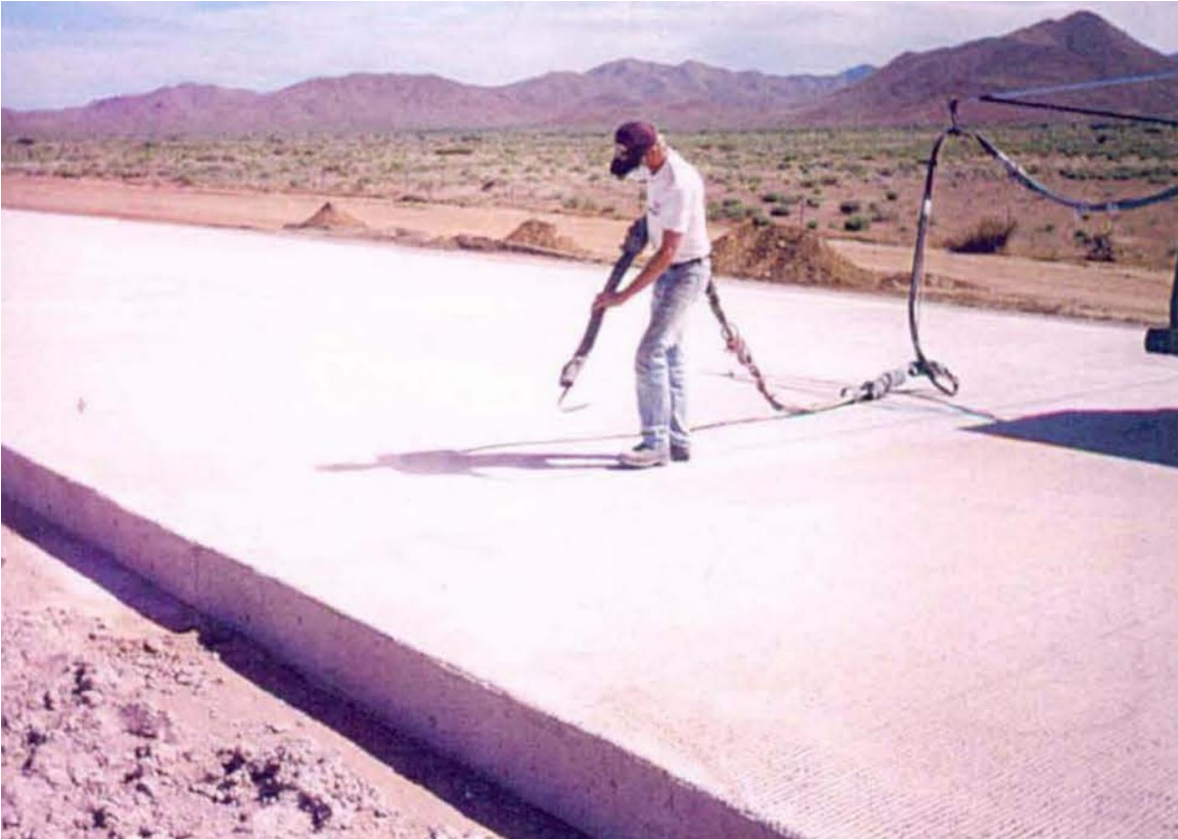
Figure 3-7 Abrasive Blasting of Joints
