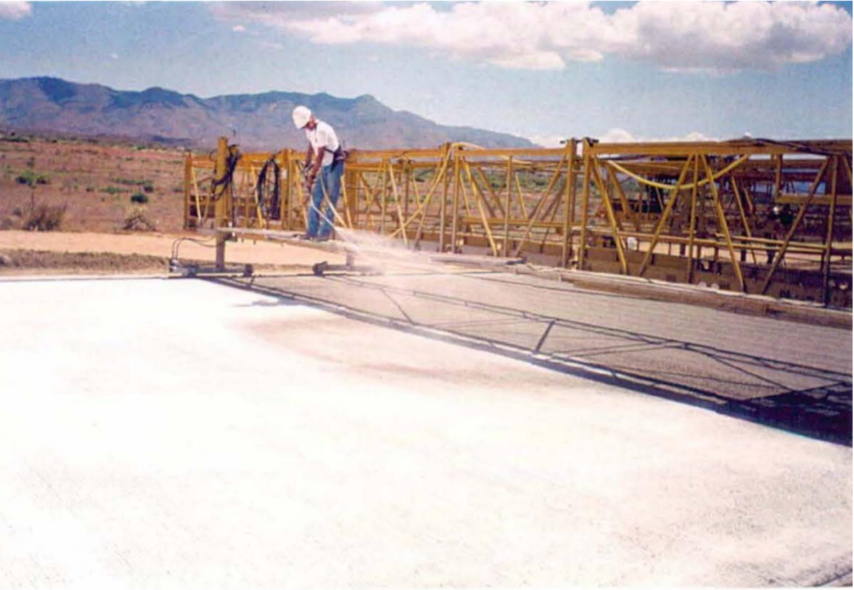
Figure 3-3 Hand Applied Curing Compound
