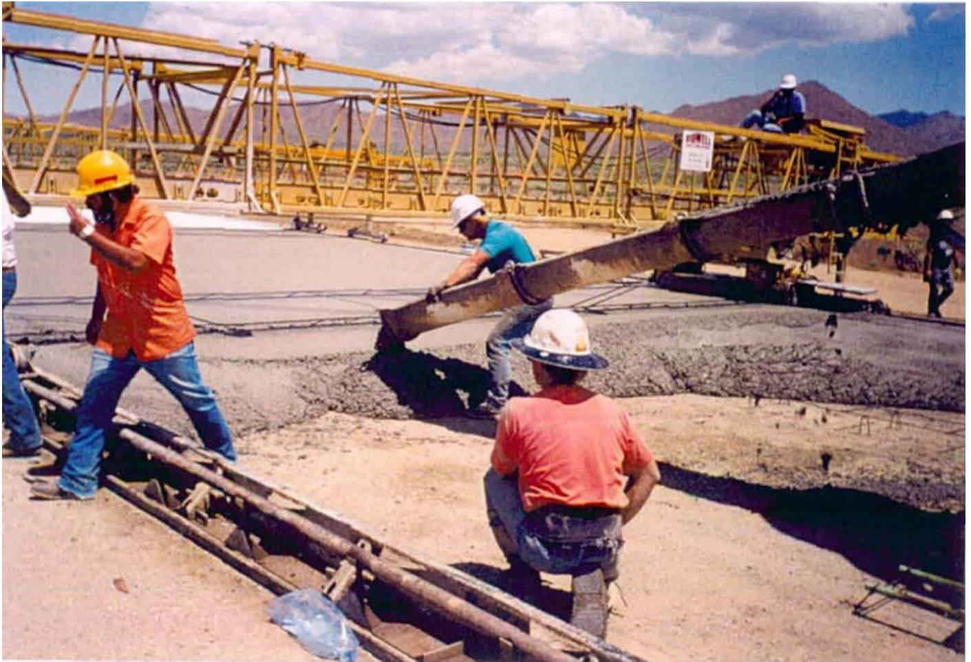
Figure 3-1 Bidwell Paving of PCCP
