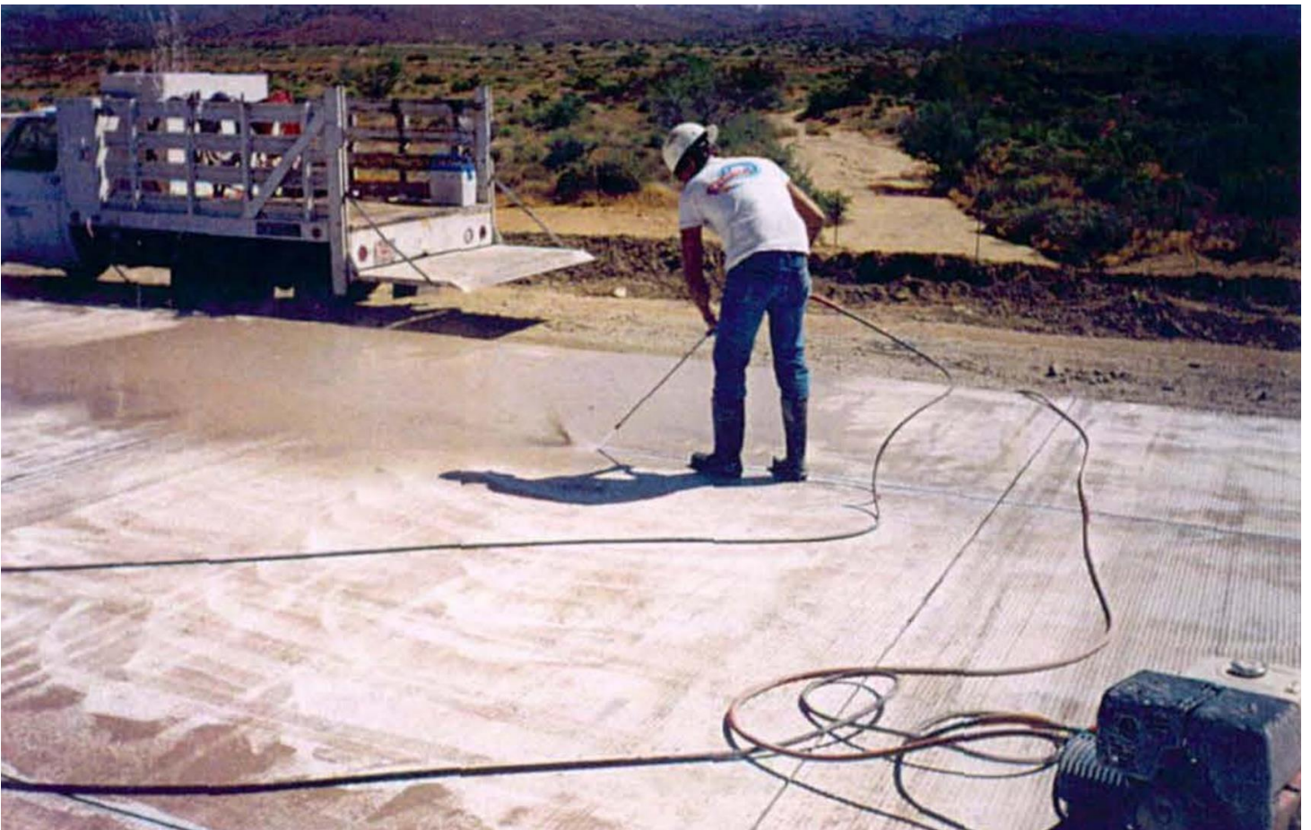
Figure 3-6 Power Washing Longitudinal Joints
