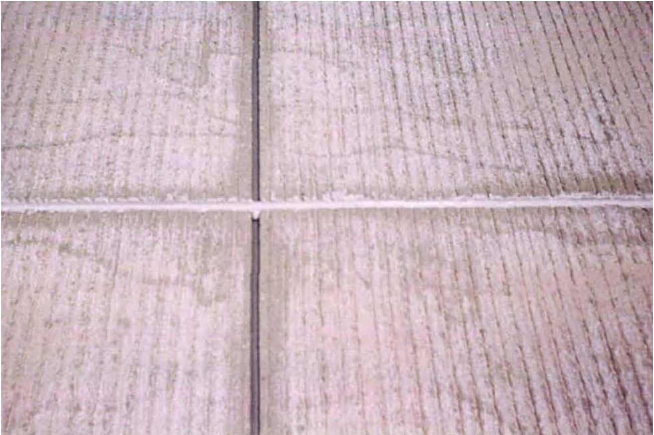
Figure 3-8 Backer Rod and Sealant Installation
